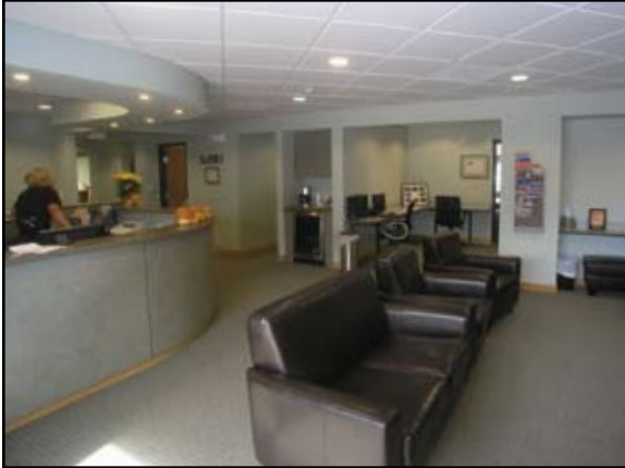
Fig. 9 Acoustical tile used in spacious reception room for noise control.
